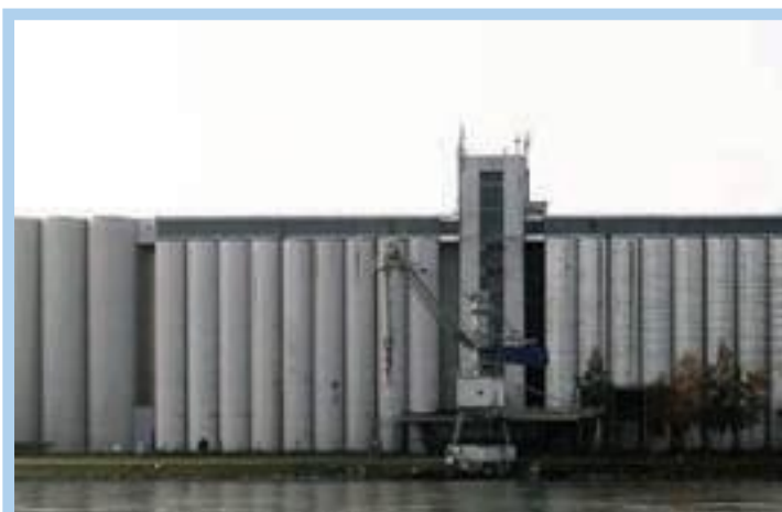
Water elevator in Zaporozhye region 100 000 tons
